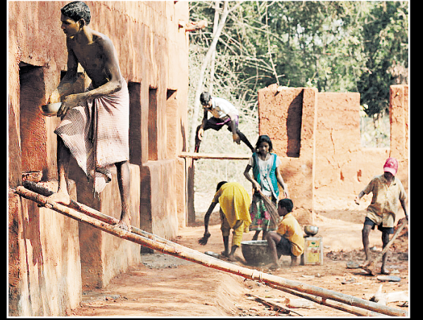
Villagers rebuild the cultural centre that was struck down by Cyclone Phailin last October
